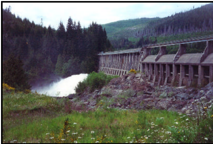
Figure 1: Jordan River Diversion Dam.
