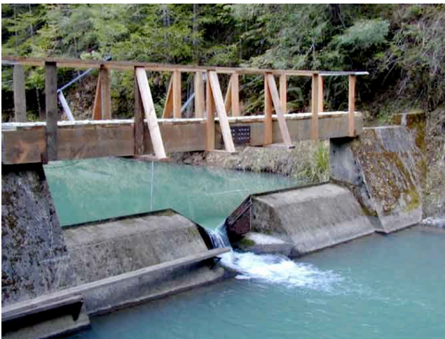
Figure 16: A man made weir for stream flow measurements
