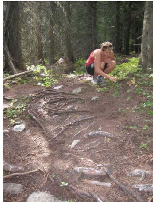
**Figure 6. Example of a wide portion of the trail with fairly severe root exposure**
