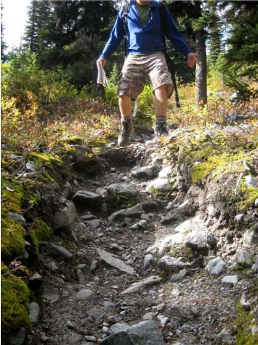
**Figure 5. Example of a severely incised portion of the trail**
