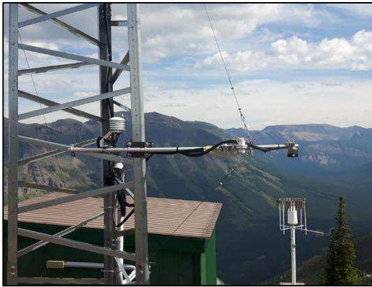
Hydrometeorology equipment at West Castle
