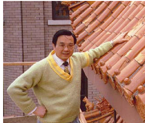
{David Lai pointing out damage in the famous Chinatown Gate of Harmonious Interest}
