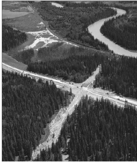
Figure 7: View east from above the upper fan on 5th August 1999, showing the debris flow deposit extending across Highway 1 to the CP Rail line adjacent to the Bow River. Five Mile Creek is being diverted into the Vermilion Lakes wetlands in the upper left of the photo.
