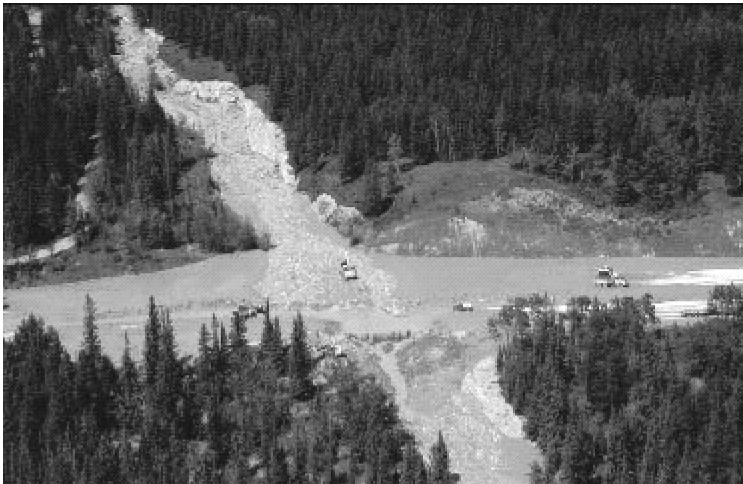
Figure 5: Highway 1 closed by the debris flow, 5th August 1999. View is upstream from above the lower fan.
