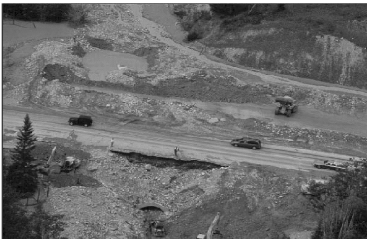
Figure 6: With the westbound lanes still buried by the debris flow deposit (top of photo) late on 5th August 1999, westbound traffic is being diverted via the eastbound lanes. The destroyed telecommunication line to Lake Louise is beneath the road edge where two individuals are standing.
