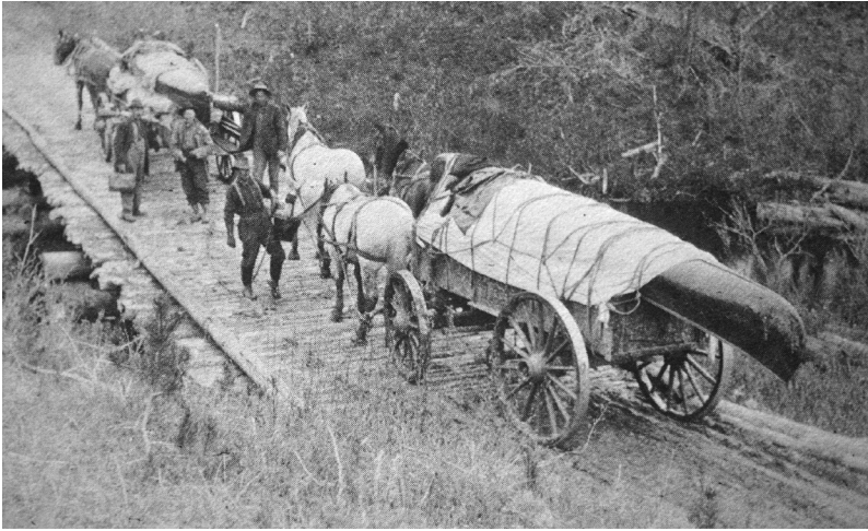
Plate 4 Wagon crossing Tay Creek bridge on the Giscome Portage, 1914 Source: BC Forest Service
